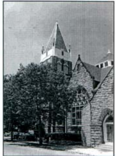
Structural and Ornamental Sheet Metal, First United Methodist Church, London.
